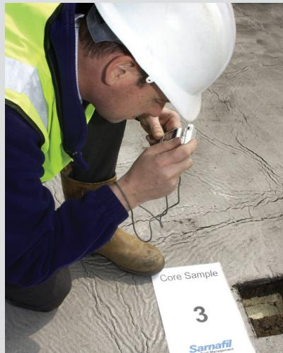
The existing roof construction and insulation were confirmed by taking core samples for analysis.
