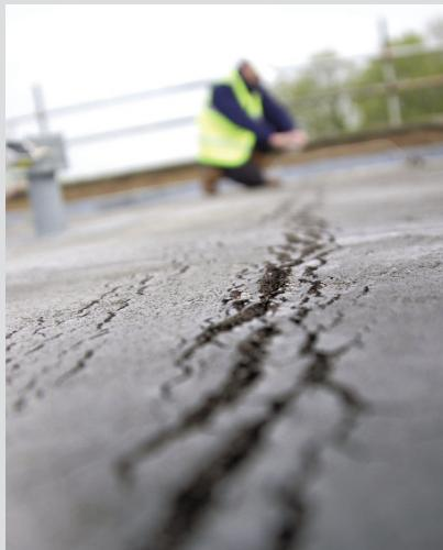
The existing asphalt roof had slumping, incorrect detailing, blisters and cracks in the asphalt, and insulation that no longer met current regulations.
